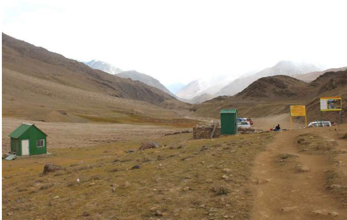
Image 11: Newly constructed toilet and guard room at Chandertal parking.
