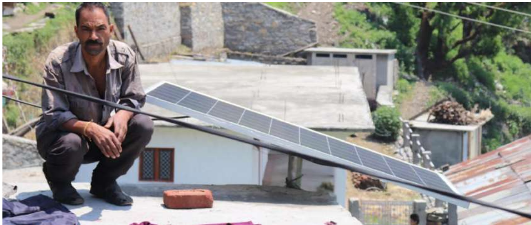
Figure 5: UPCL provided and self-installed solar PV home system in Tihar village
